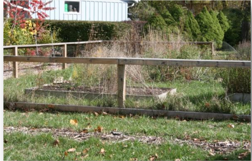
This garden is protected using chicken wire framed with 2"x4"s attached to 4"x4" posts. The height is 4 feet, enough to keep cottontails out and to stop casual foraging by deer.
