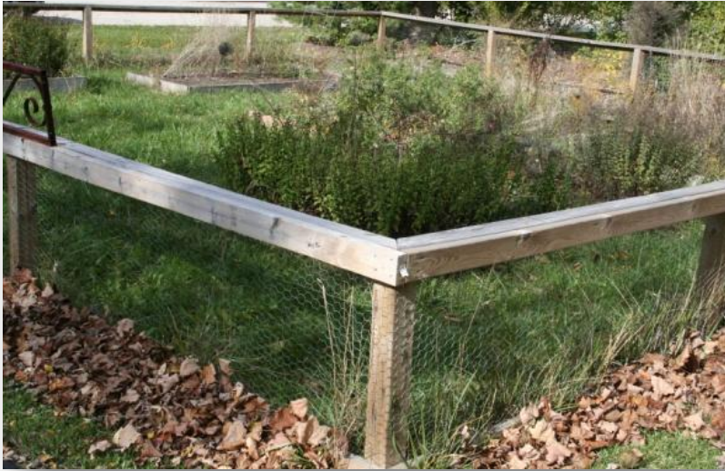
This garden is protected using chicken wire framed with 2"x4"s attached to 4"x4" posts. The height is 4 feet, enough to keep cottontails out and to stop casual foraging by deer.
